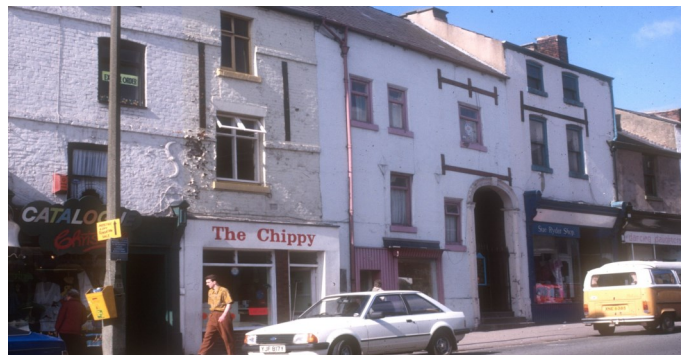
St. Mary's entrance and associated buildings. 1986
