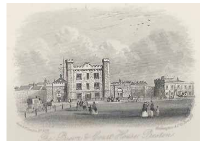
The Prison and Court House, Preston, 1856.
