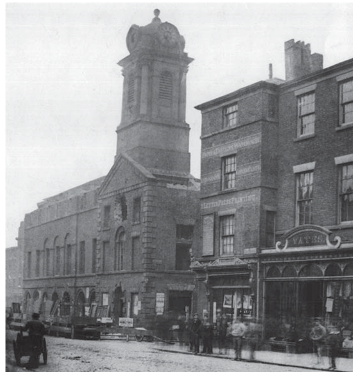
Preston's 'Old' Town Hall in the process of being demolished in 1861.
