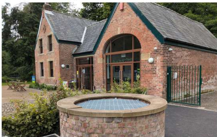
Hurst Grange Coach House showing reconstructed well in the foreground. With no running water, the well was the water supply for the coach house and gardens.
